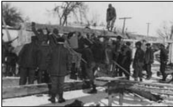
*Men were working on hemlock 12"x 12" beams, 12 feet in length. Five beams were joined by tenons and pegs to make the 60 foot beams. The narrow diagonal poles were set up on both sides of the beam and were used by the men to elevate the beam.*
