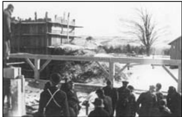
*In the foreground, a "bent" was prepared: a tie beam, posts, and braces. Wooden pegs were used as joinery. In the background, a square wooden silo was begun; it was since torn down and replaced.*
