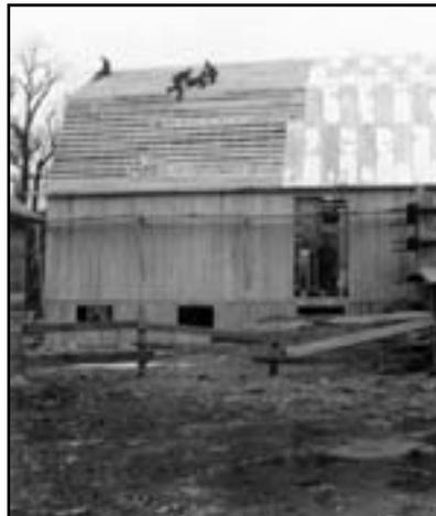
*Men were working on roofing. Rafters and nailing strips were exposed on the left, and metal roofing was installed on the right. The roofing was periodically painted and is still in use.*
